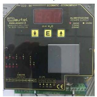
Economisers in the ECOMATIC-S range are digital sequential timers with built-in differential pressure switches.
