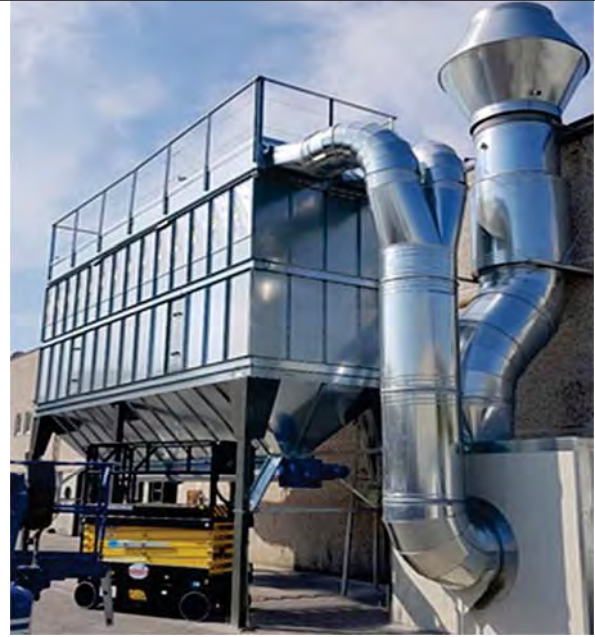
BERF 42 120 2500 1 T with screw and extraction fan in acoustic booth
